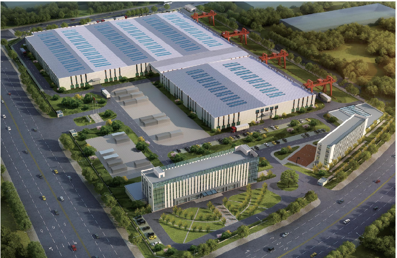
An Annual Output of 100,000 Sets of High-end Slewing Ring Intelligent Production Plant
